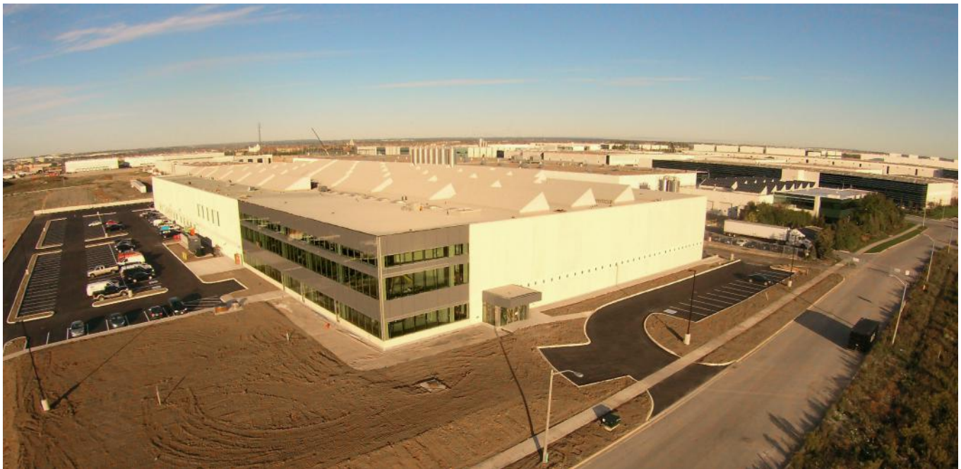
Photo of new 155,000 sq ft Systems Center; current Athena facility in background.
