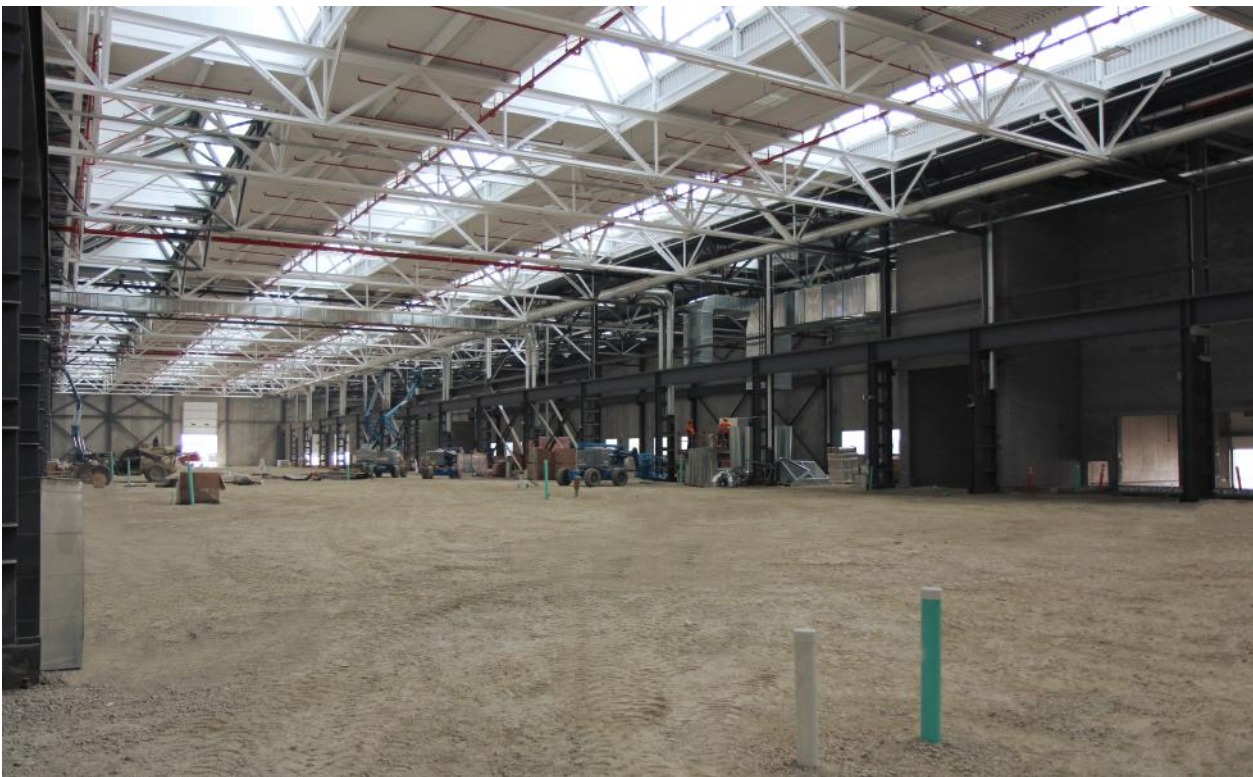
The 150 m (492 ft) long main hall; two 50-ton cranes will span its width and travel the entire length.
